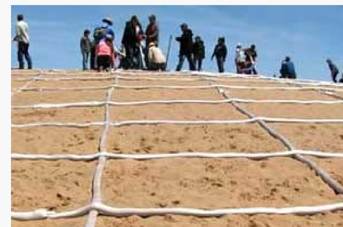
Figure 6. Illustration of the grid pattern of the sand sausages to maintain the sand dunes on the Navajo Nation
