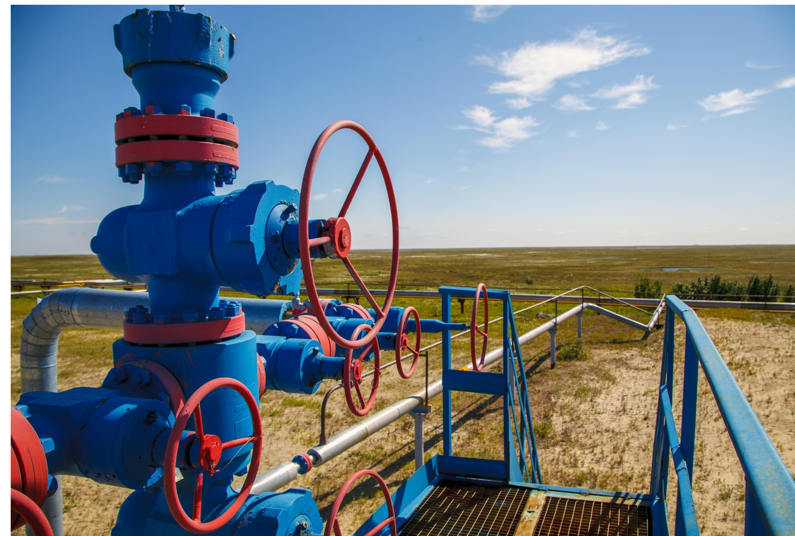
Figure 3. Oklahoma Gas Well-head Source: Oklahoma Corporation Commission
