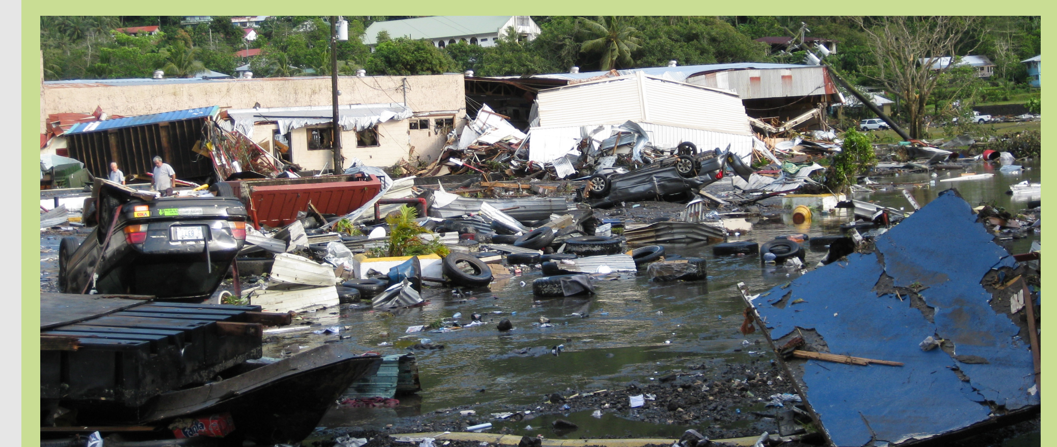
Buildings damaged in Tutuila, American Samoa after the tsunami Courtesy of NOAA NCEI/Gordon Yamasaki
